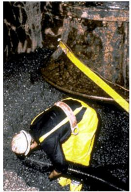
Worker removing zebra mussels from water intake pipes.
